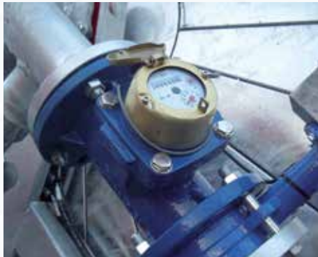
Flanged litre-counter on reel inlet.
